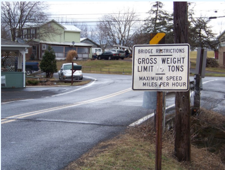
Site of upcoming bridge reconstruction project at Snook's Hill Road in Granville Township.
