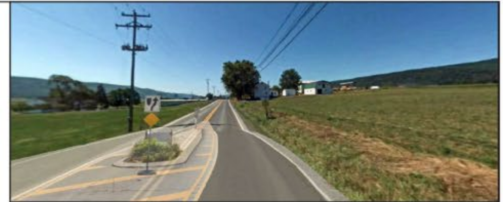
Gateway medians at east and west ends of Allensville to calm traffic.
