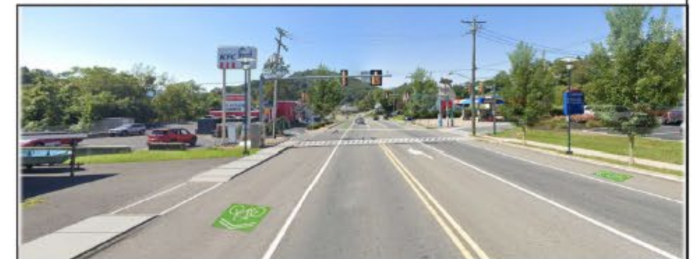
Sidewalks and intersection crosswalks at 3rd Street and 4th Street to provide access to destinations on South side of SR 1105/ Electric Avenue.
