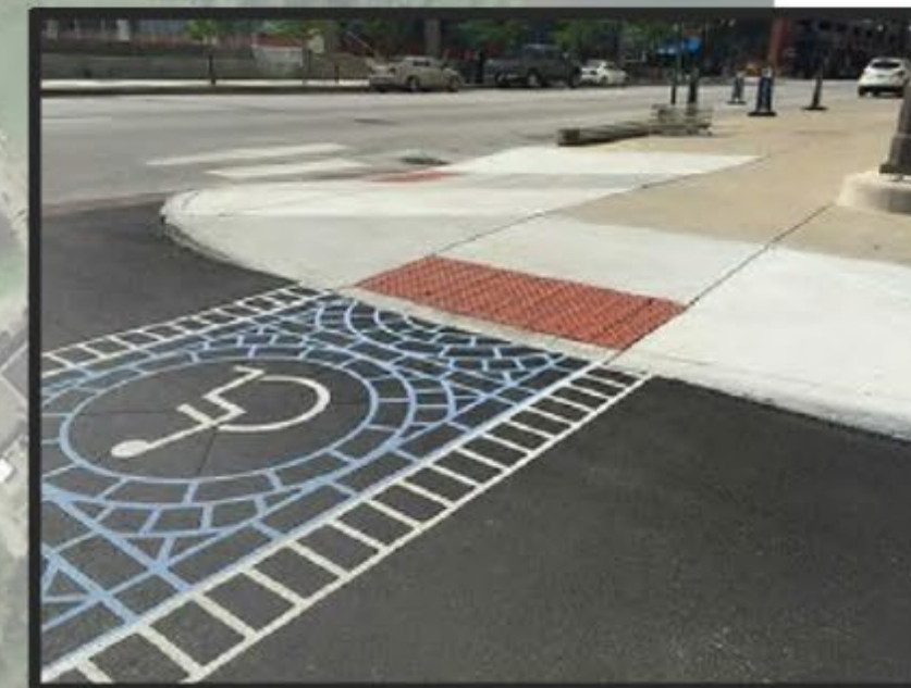
ADA SITE IMPROVEMENTS
