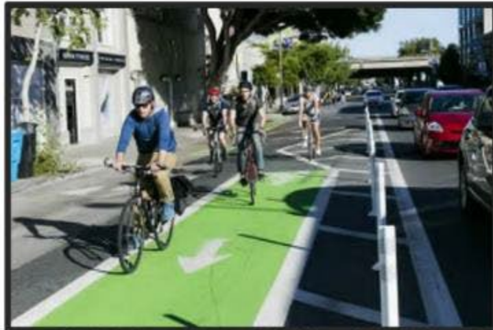
PEDESTRAIN/BIKE PATH IMPROVEMENTS
