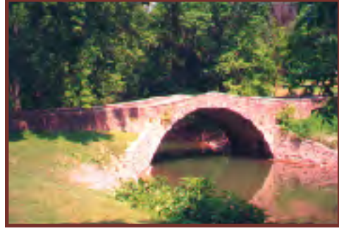
STONE ARCH BRIDGE
