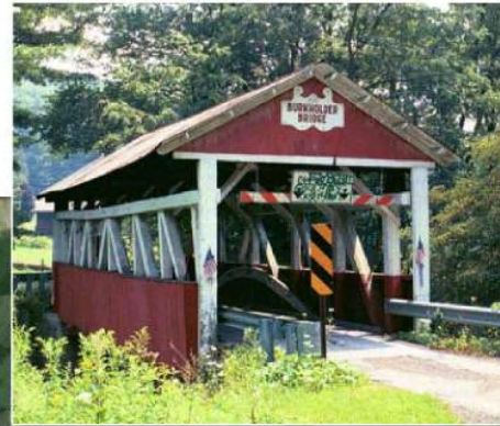
Existing historic 1870 Burkholder Covered Bridge (Excellent Condition)
