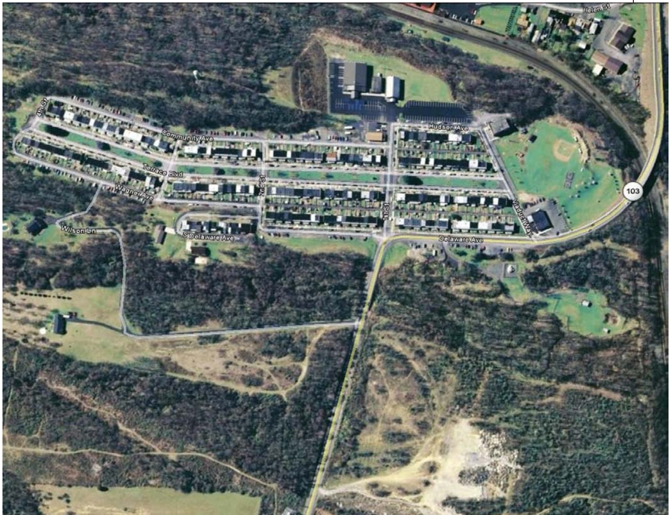
Figure C.15. Aerial View of Juniata Terrace
