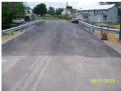
Final bridge surface
