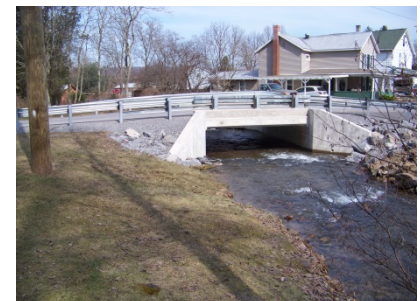
Final Bridge after construction
